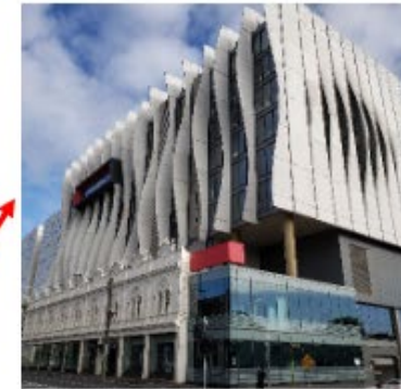
AMDC Building Level 5
